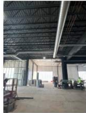
Ductwork being installed in lobby ceiling
