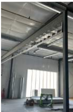
Track for divider curtain installed
