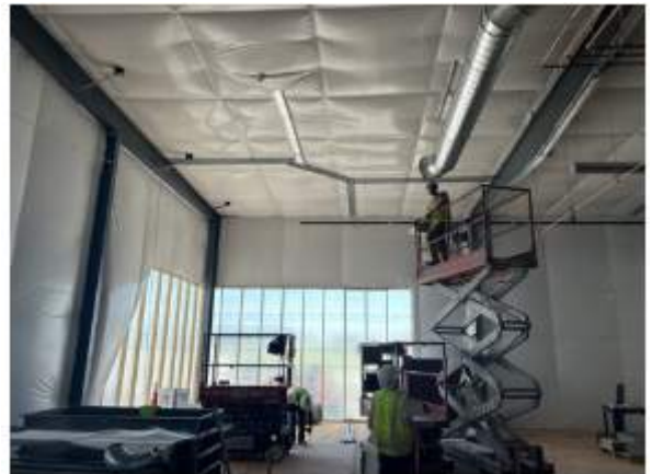
Top track installation on North side
