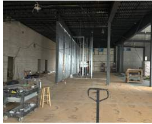
Shower room stud installation
