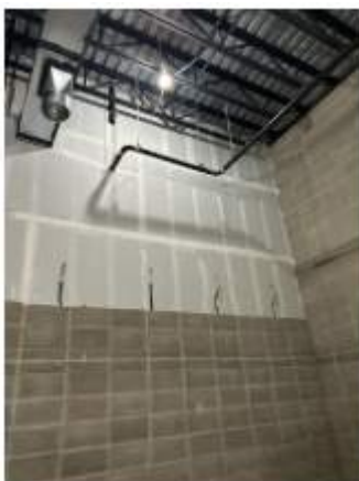
Locker room drywall installation
