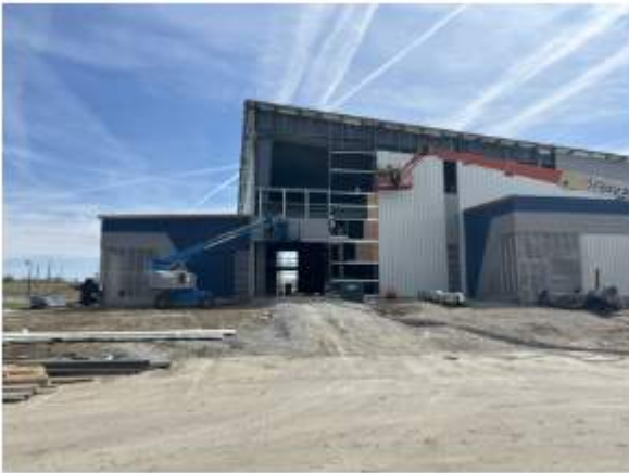
West side metal panels wrapping up
