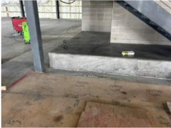
Concrete bench poured
