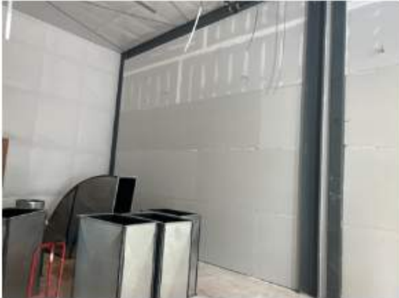
Mechanical room drywall installation
