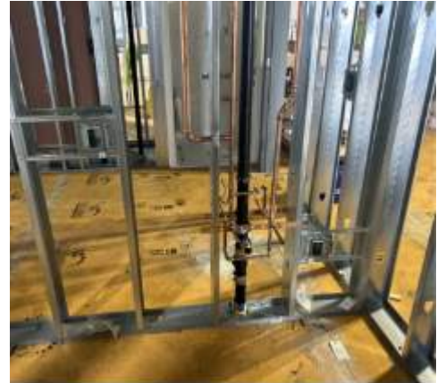
Sink installation in shower rooms
