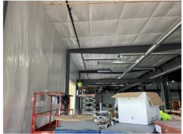
Ductwork & Fire Protection installation on North side
