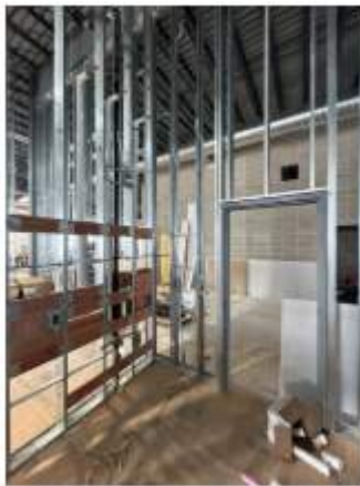
Additional blocking and rough-in in shower rooms
