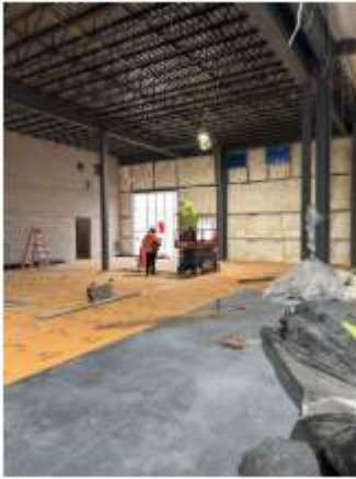
Shower room walls being laid out
