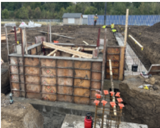
Elevator walls and locker room footings poured
