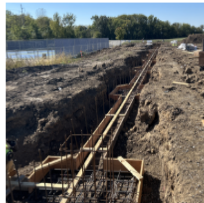
Grid Line F footing formed
