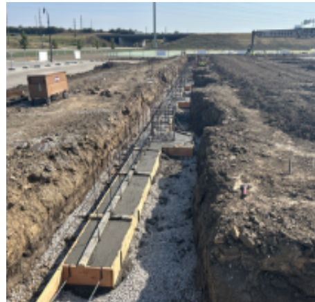
Grid Line A footing poured
