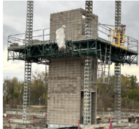
Elevator shaft just over 2 nd floor door opening
