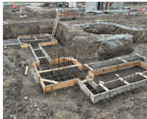
Grid Line A and front stoop footing formed
