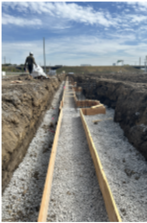
Grid Line A footing formed
