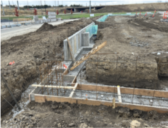
Grid Line 1 and Grid Line 11 foundation walls poured, insulated, and starting to backfill
