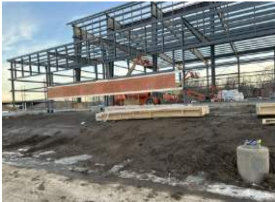
Backing installed for North building sign
