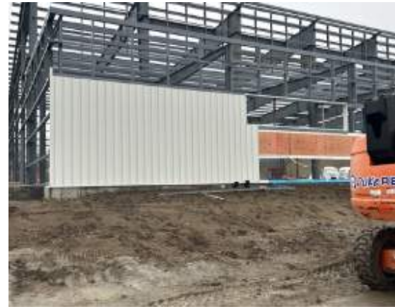
First exterior metal panels being installed
