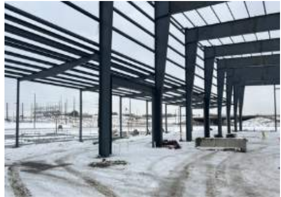
North side roof purlins
