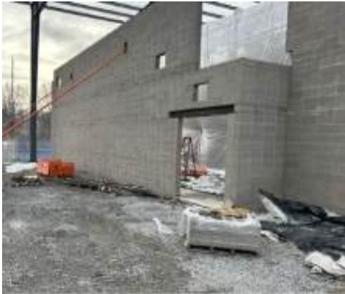
East locker room CMU wall complete
