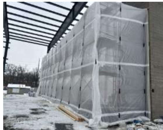
East locker room CMU wall starting
