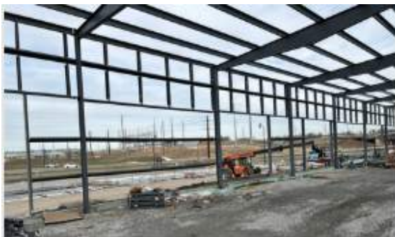
North building girts and jambs being installed
