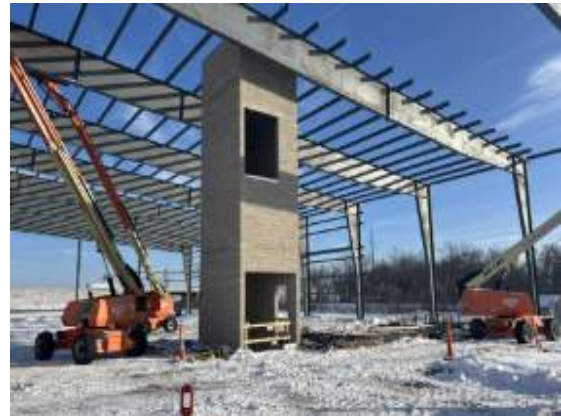
Continuation of roof purlins
