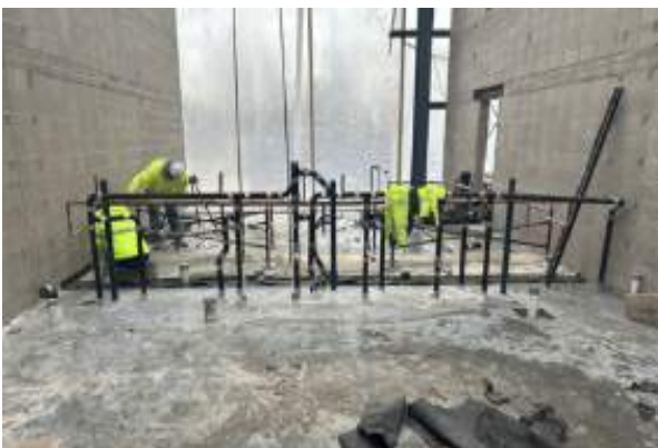
East and West locker room CMU walls complete. Plumbing inside chase wall and layout of interior CMU walls
