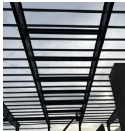
Steel for track installed
