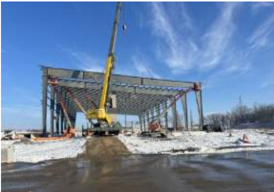
Last PEMB beam for the court area
