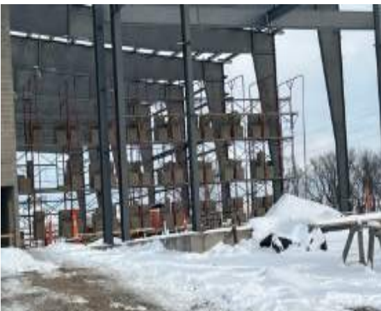
Mason's preparing for East locker room wall
