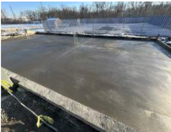
Southwest mechanical pad poured
