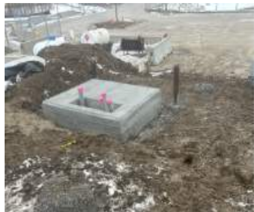
Transformer pad complete
