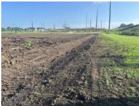
Placement of topsoil looking North
