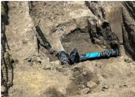
Water main tied into main line
