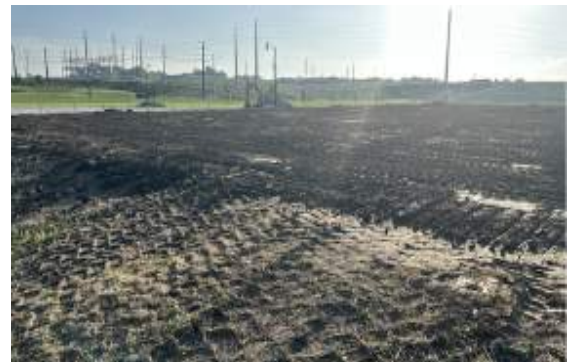
Surcharge stripped off building pad
