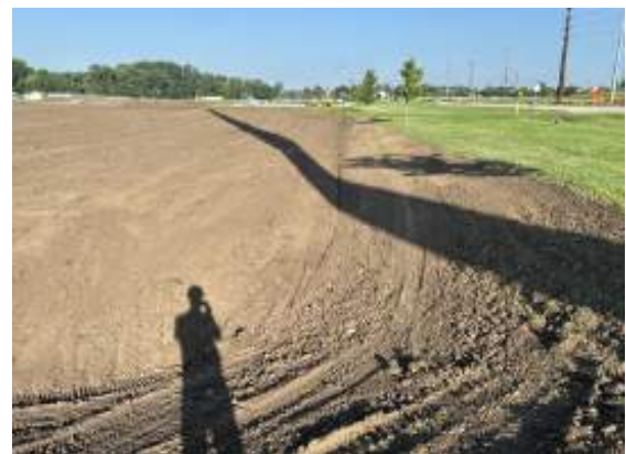
Placement of topsoil looking West
