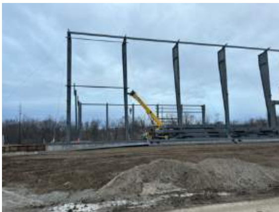
Columns standing along GL B and F
