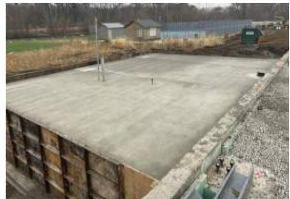
Southeast mechanical pad poured
