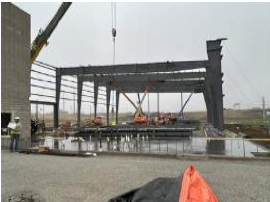
Installing beam along Grid Line 8
