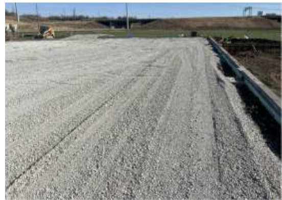
Rock subbase being installed and leveled out
