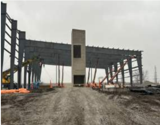
PEMB looking east with 6 beams installed
