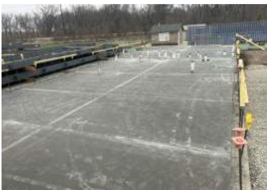
Locker room slab on grade poured and cut
