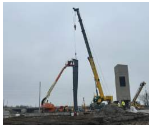
Installation of first PEMB column
