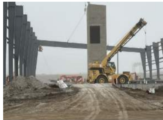
First beam being installed along Grid Line 11
