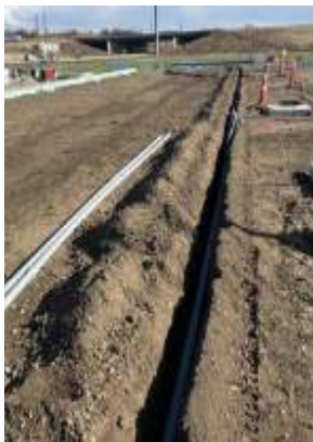
Underground electrical being installed to the East
