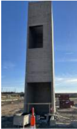
Elevator shaft is complete
