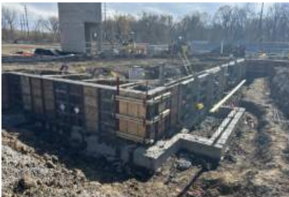
Last foundation wall being poured
