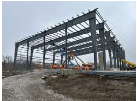
Installing roof girts
