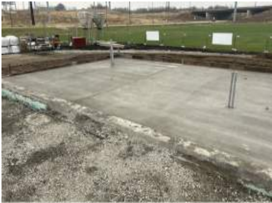
Northeast mechanical pad poured
