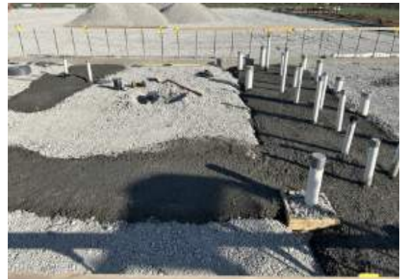
Thickened slabs under interior CMU walls poured
