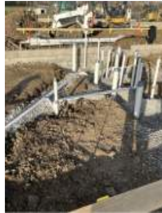
Installation of underground plumbing in locker rooms
