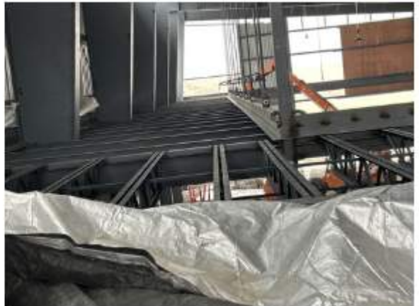
Track steel being installed along the North
