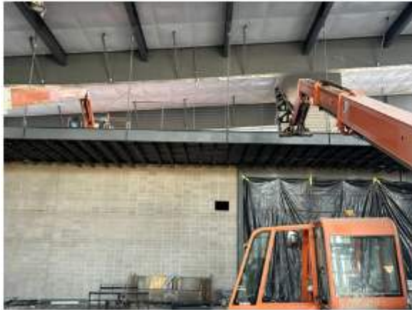
First section of handrail being installed around track
