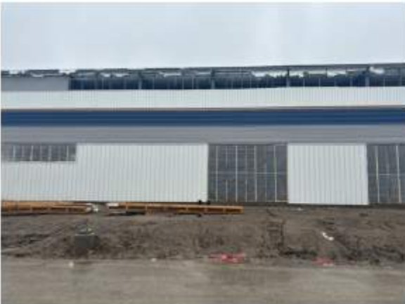
Exterior metal panel progress with the blue accent color
