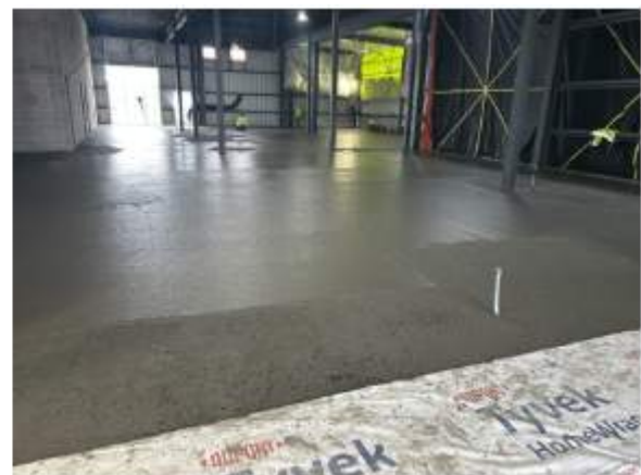
Slab on grade pour by entrance and shower rooms
