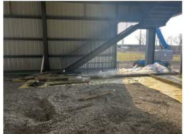
East gym stair installed with handrail
