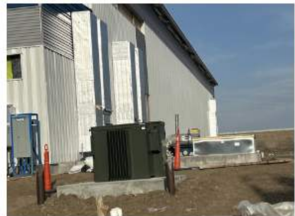
Southwest and Southeast duct installed
