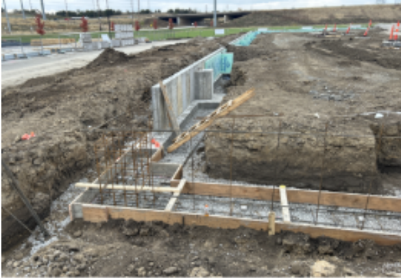
Grid Line 1 and Grid Line 11 foundation walls poured, insulated, and starting to backfill
