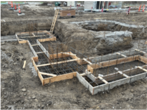
Grid Line A and front stoop footing formed
