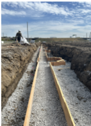
Grid Line A footing formed
