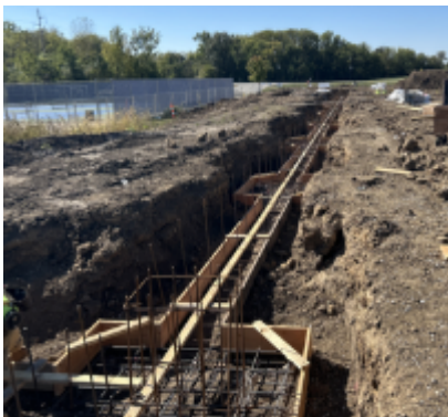
Grid Line F footing formed
