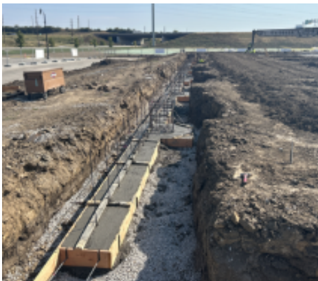
Grid Line A footing poured
