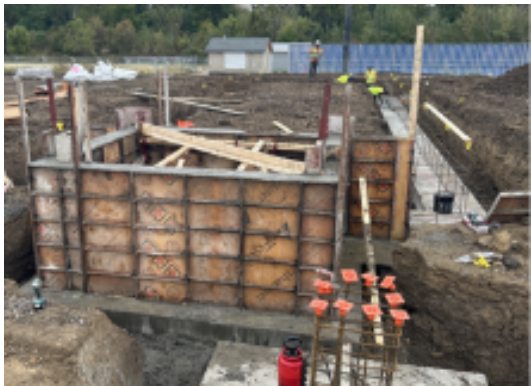
Elevator walls and locker room footings poured
