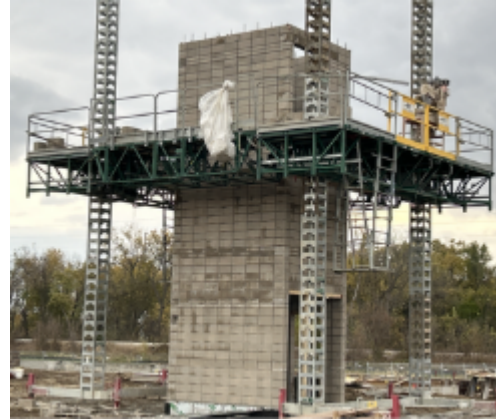
Elevator shaft just over 2 nd floor door opening
