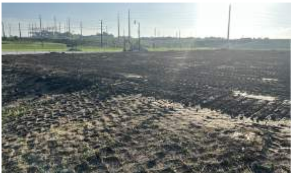
Surcharge stripped off building pad
