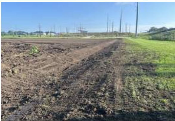
Placement of topsoil looking North
