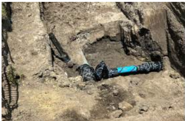
Water main tied into main line
