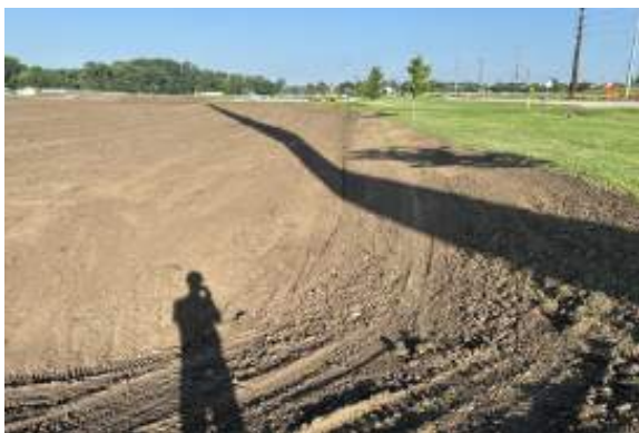
Placement of topsoil looking West
