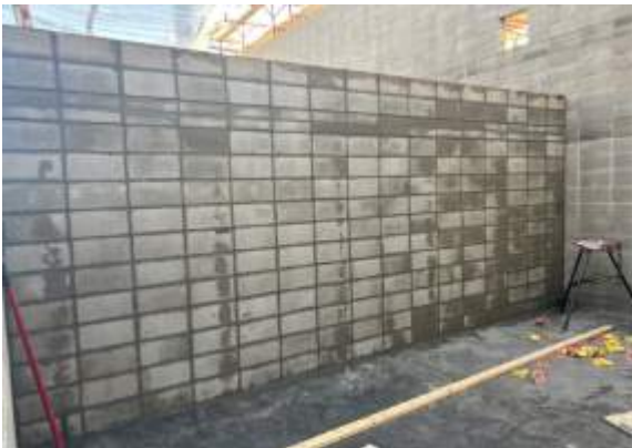
Storage room CMU wall completed
