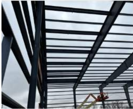
High steel for running track being installed
