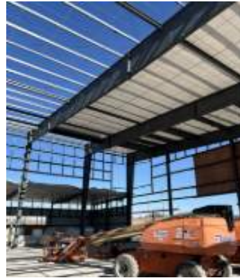
First roof liners being installed in high bays
