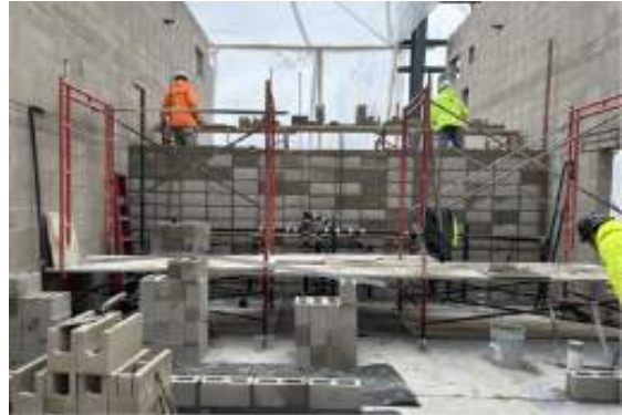
Interior CMU walls being installed (Plumbing chase)
