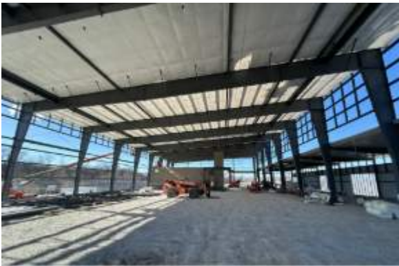
Roof liner along with roof insulation in high bays
