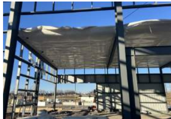
Building B Roof being installed
