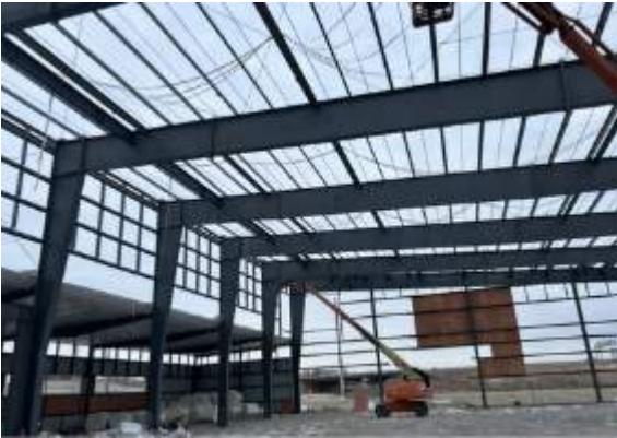
Strapping for roof liner being installed in high bays
