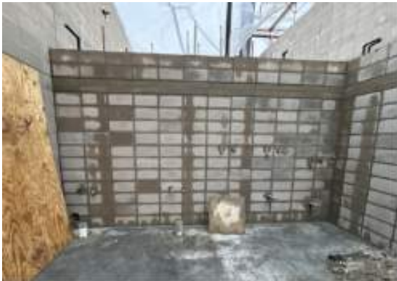
Men's Locker room plumbing chase completed
