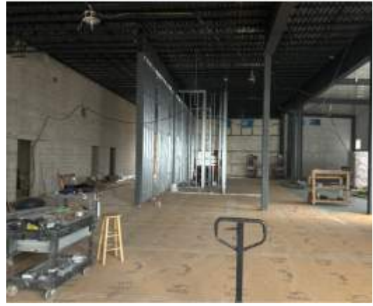
Shower room stud installation
