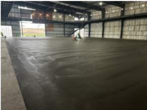
Gym floor poured and being finished
