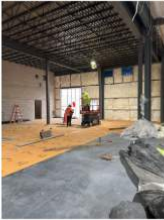
Shower room walls being laid out
