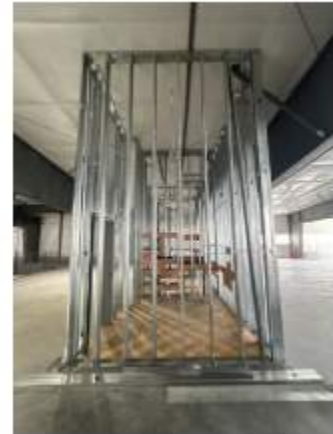
2 nd Floor in wall rough-ins and blocking
