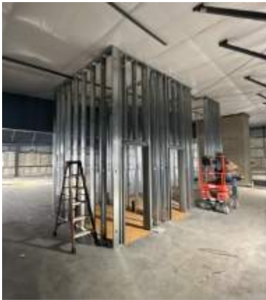
2 nd Floor stud installation
