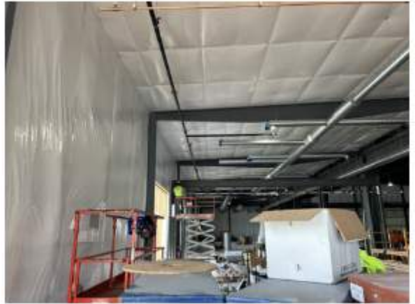
Ductwork & Fire Protection installation on North side
