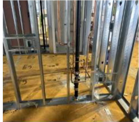
Sink installation in shower rooms
