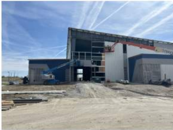
West side metal panels wrapping up
