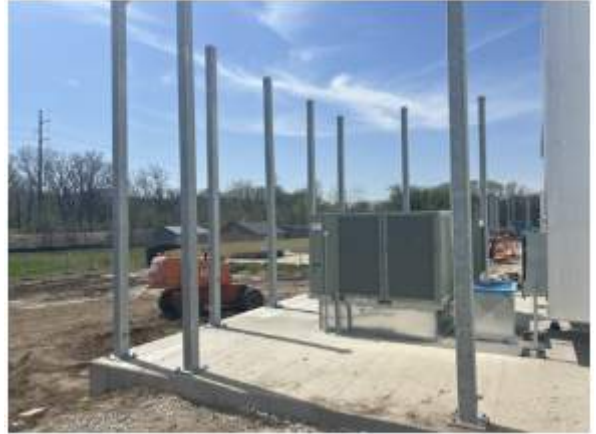
Screen wall columns being installed
