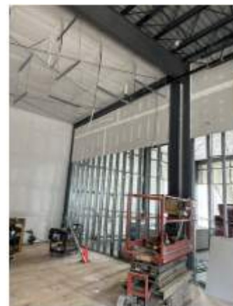
Mechanical room drywall installation
