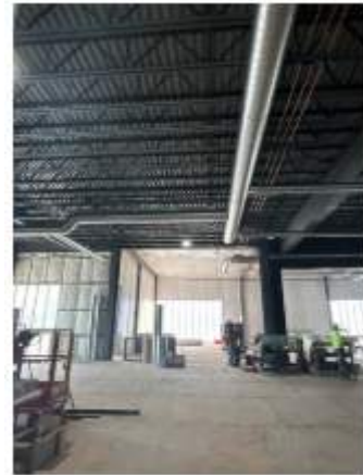
Ductwork being installed in lobby ceiling
