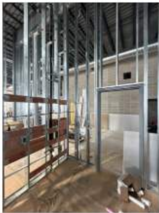
Additional blocking and rough-in in shower rooms
