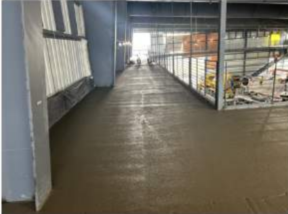
Concrete on track looking East
