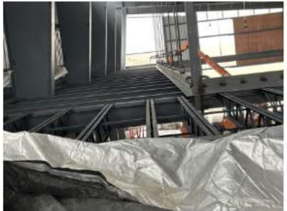
Track steel being installed along the North
