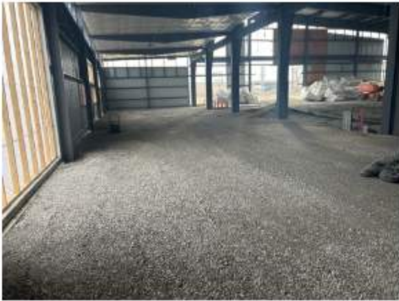
Prepping slab on grade. Looking East towards turf room
