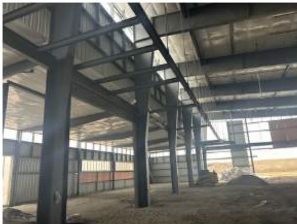
Prepping slab on grade
