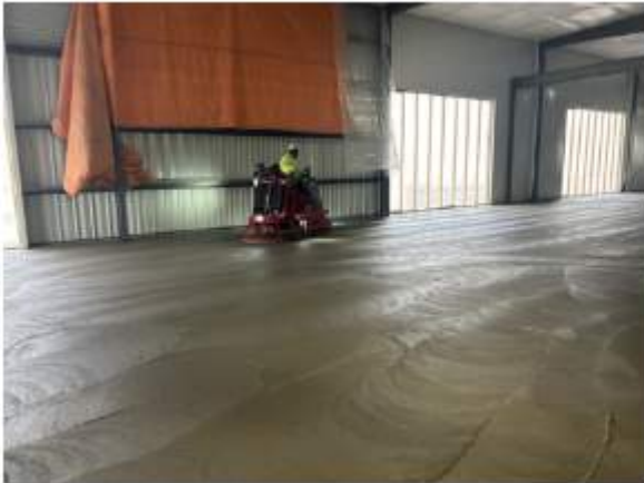
Concrete finisher by studio rooms
