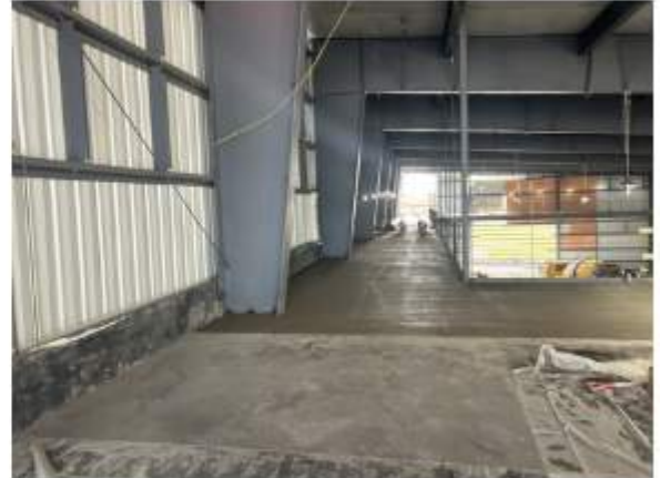
Last pour of 2 nd floor, concrete on track
