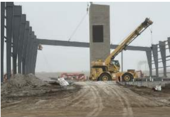
First beam being installed along Grid Line 11
