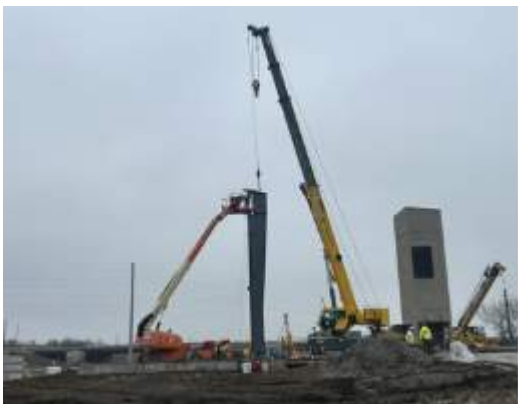
Installation of first PEMB column
