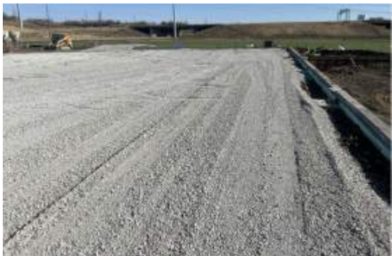
Rock subbase being installed and leveled out
