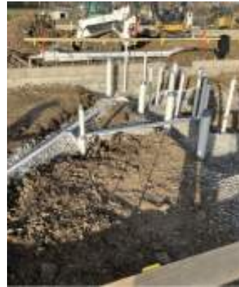
Installation of underground plumbing in locker rooms
