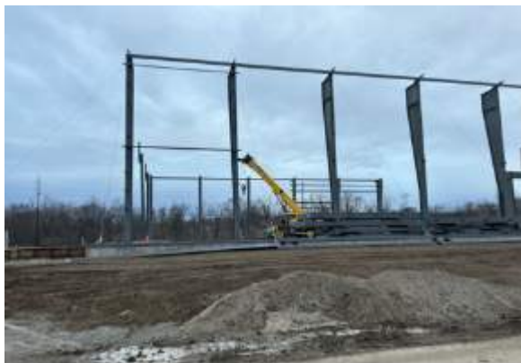
Columns standing along GL B and F
