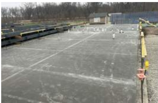
Locker room slab on grade poured and cut
