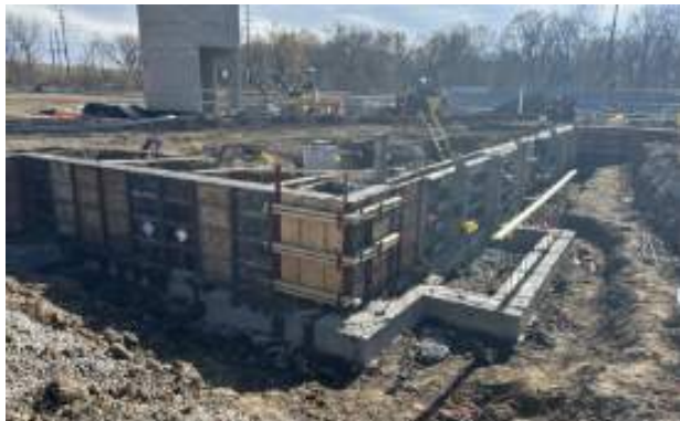
Last foundation wall being poured
