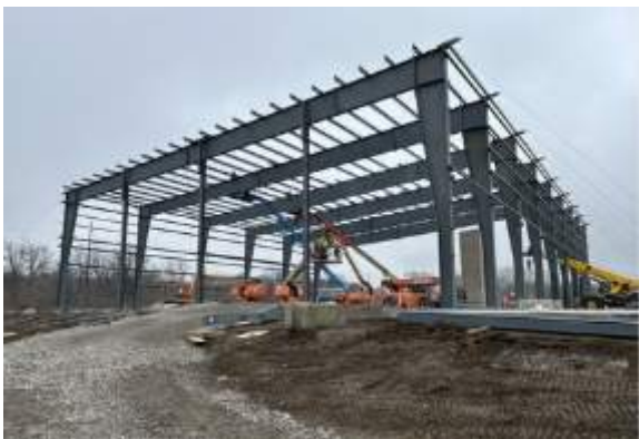
Installing roof girts
