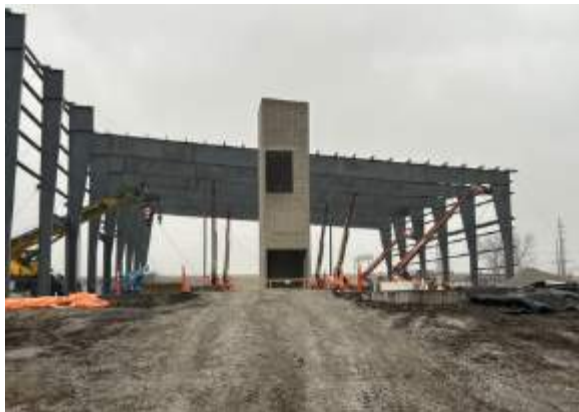
PEMB looking east with 6 beams installed
