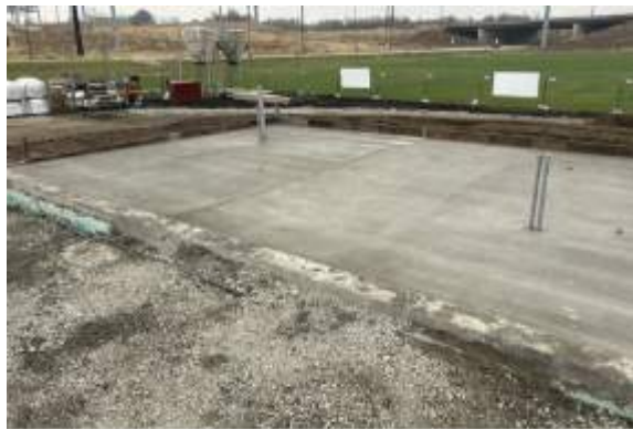
Northeast mechanical pad poured
