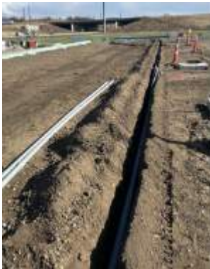
Underground electrical being installed to the East
