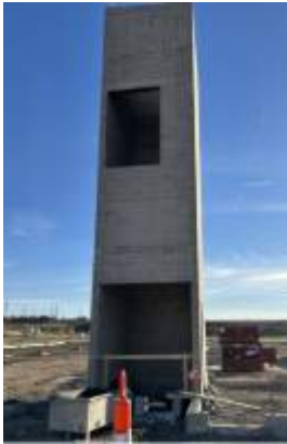
Elevator shaft is complete
