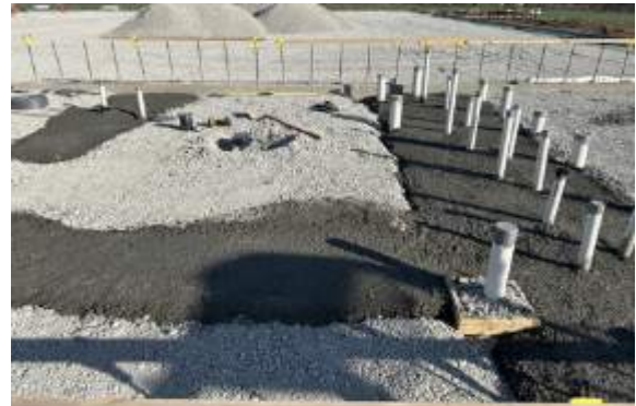
Thickened slabs under interior CMU walls poured
