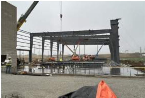
Installing beam along Grid Line 8
