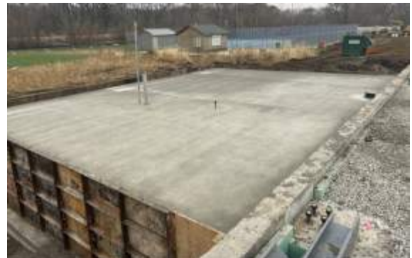
Southeast mechanical pad poured
