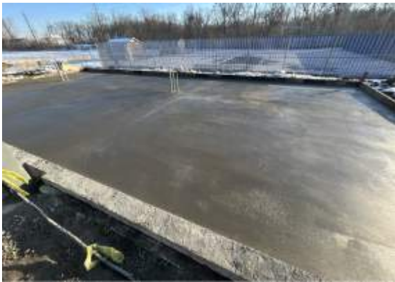
Southwest mechanical pad poured
