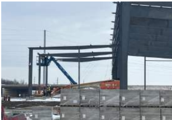
Start of North section PEMB
