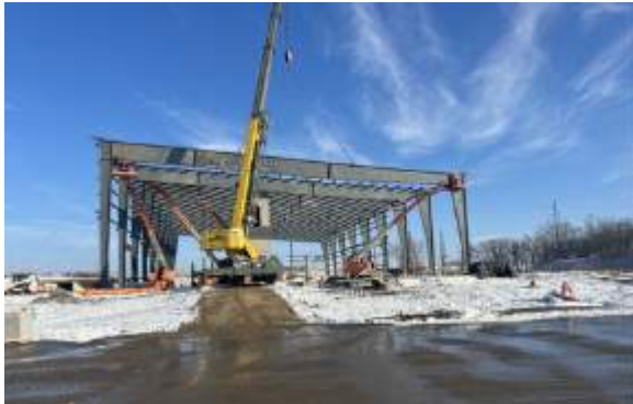
Last PEMB beam for the court area
