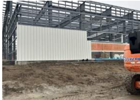
First exterior metal panels being installed
