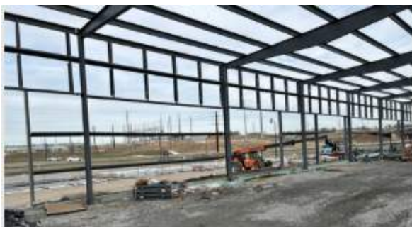
North building girts and jambs being installed
