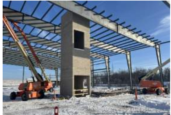
Continuation of roof purlins
