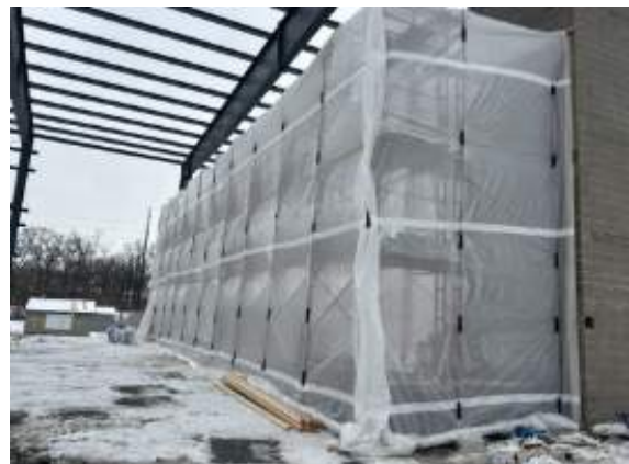
East locker room CMU wall starting
