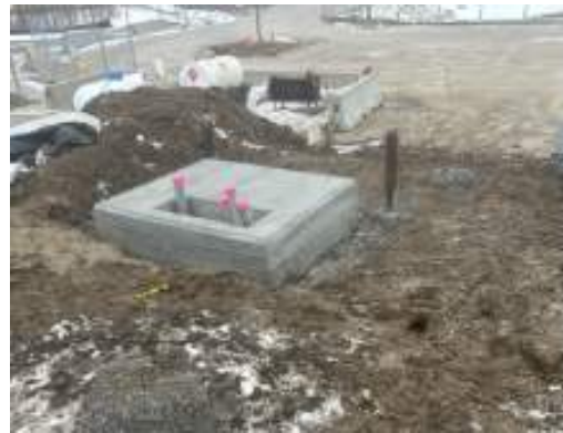
Transformer pad complete
