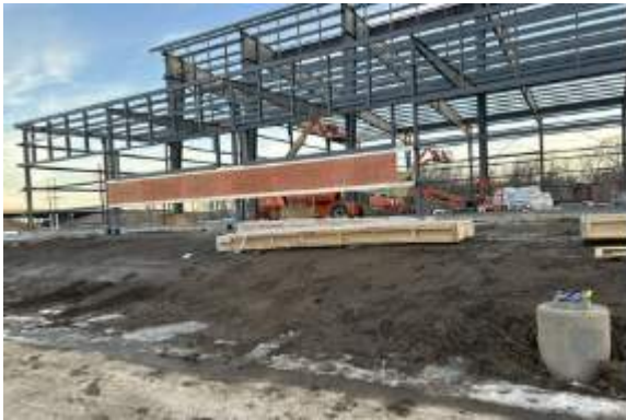
Backing installed for North building sign
