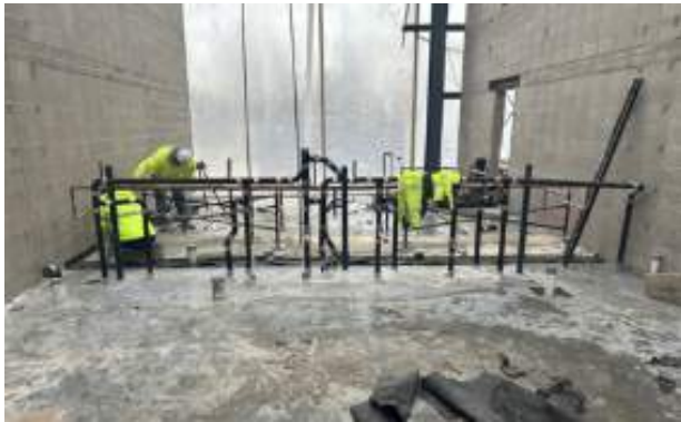
East and West locker room CMU walls complete. Plumbing inside chase wall and layout of interior CMU walls
