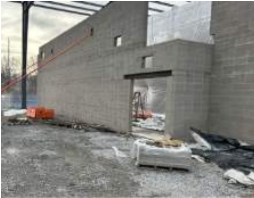
East locker room CMU wall complete
