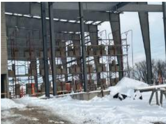
Mason's preparing for East locker room wall
