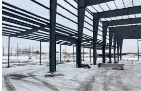
North side roof purlins
