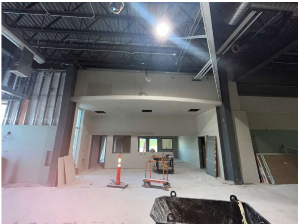
Reception desk drywall hung
