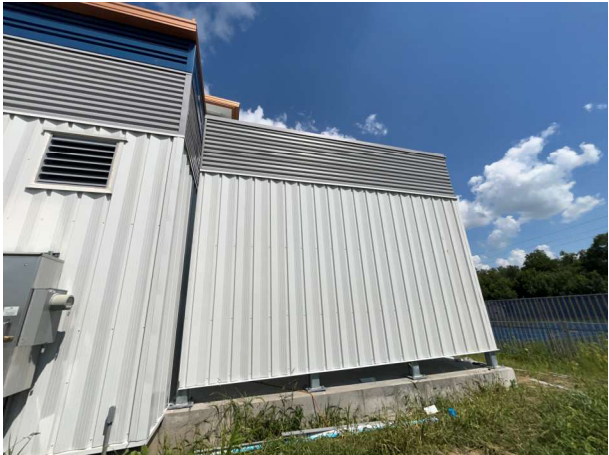
Mechanical screen metal panel install
