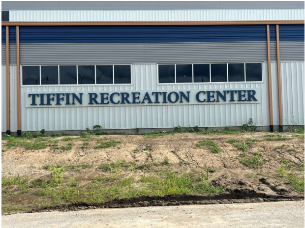
Exterior sign install
