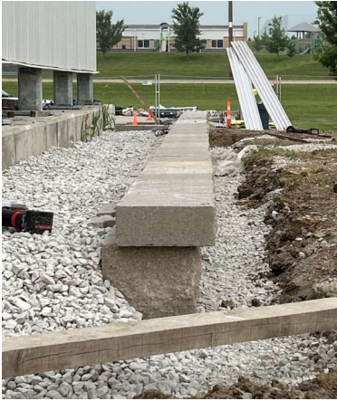
Retaining wall install
