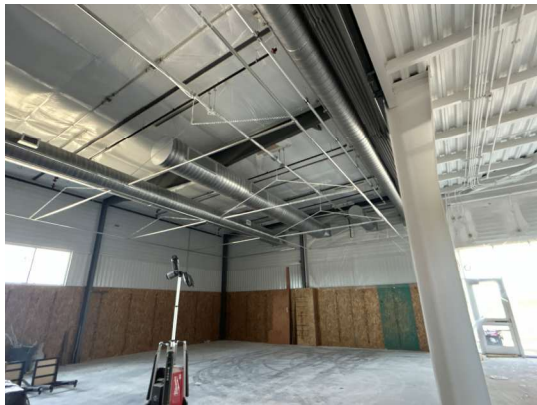
Batting cage install
