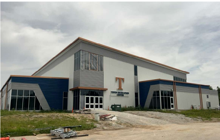
Storefront curtain wall install
