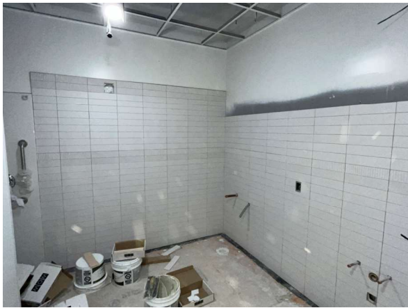
Shower room tile install
