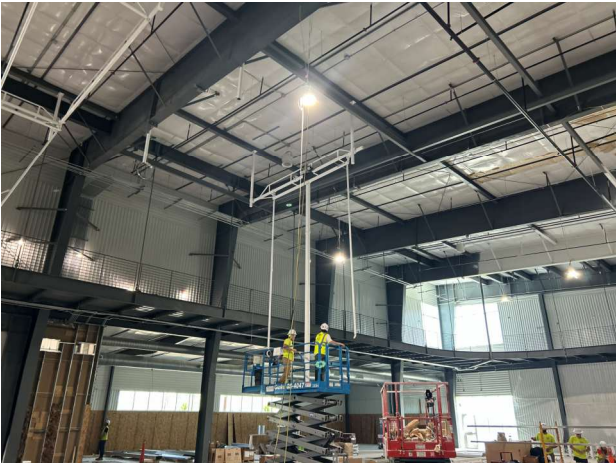
Gym equipment install
