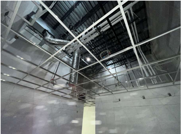
Ceiling tile grid install
