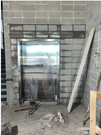
Masonry install around elevator
